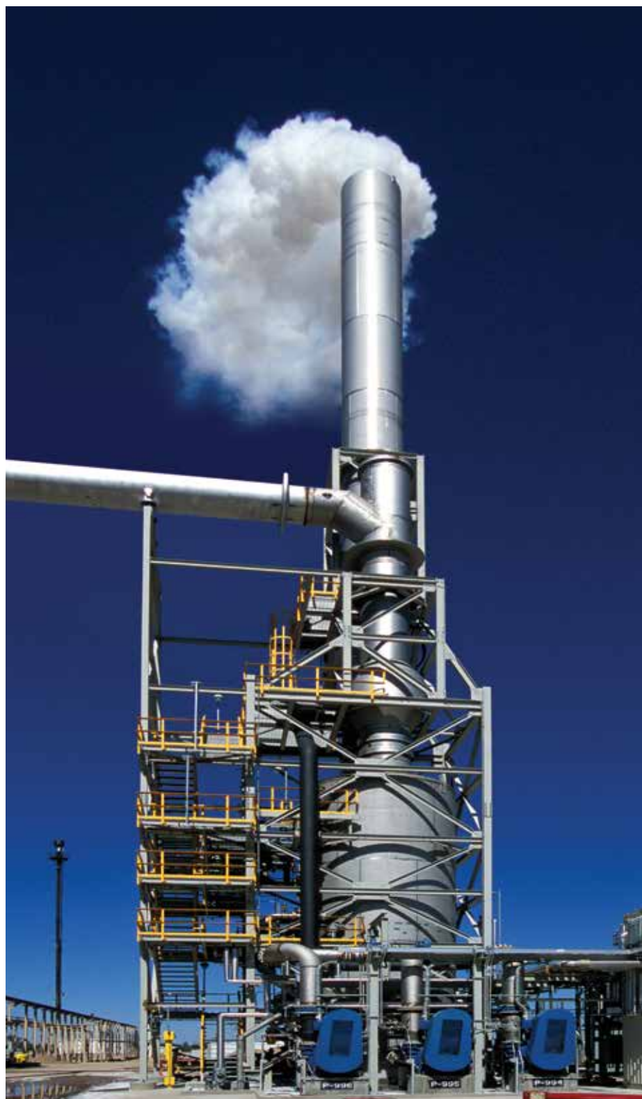
FIG. 1. The DynaWave wet scrubbing technology is a Claus tail gas treatment unit (TGTU) supplement that makes it possible to fully bypass the unit directly to the incinerator and still meet emissions limits at the stack.
