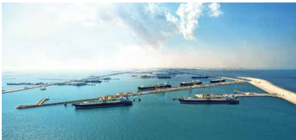
FIG. 1. Qatar's Ras Laffan port area features a CCA that is connected to all six LNG berths in the area through a 60-in. collection header.
