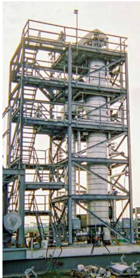
FIG. 1. The modularized D'GAASS sulfur degassing unit can successfully enhance the degassing capacity of the refinery without modifications to the existing sulfur pit.
